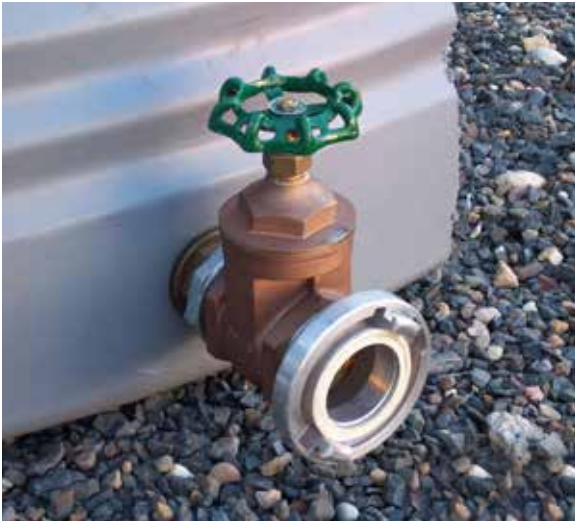
Figure 8. Gate Valve
